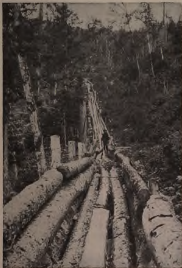
FIG. 68. — A Timber Chute. New Hampshire.
